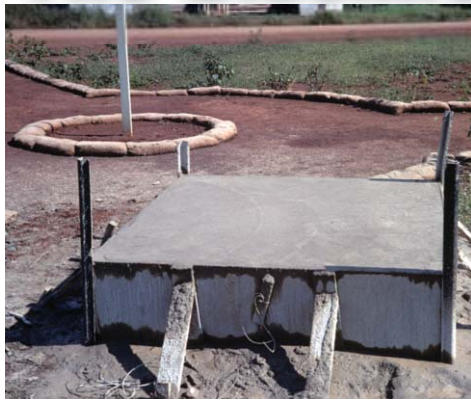
Vietnam, Blackhorse Base Camp, fall of 1967, foundation for memorial is poured.
