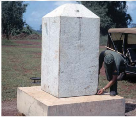
Fall of 1967, construction phase.
