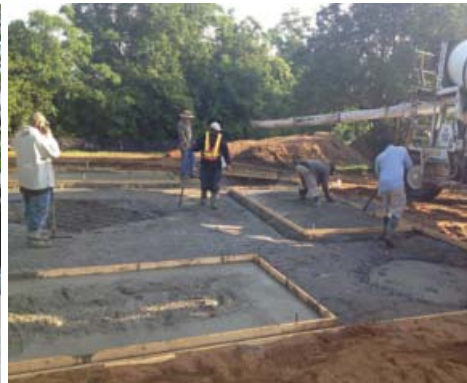
2015 pouring foundation at Ft. Benning.
