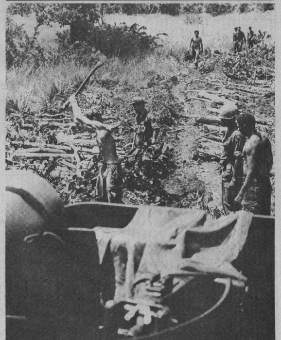
CORDUROY ROAD —Blackhorse Troopers from 2nd Squadron's G Troop encountered an old enemy, mud, while returning to FSB Marge. They reached back into history for a solution to the problem and constructed a log road. (Photo by Smith)
