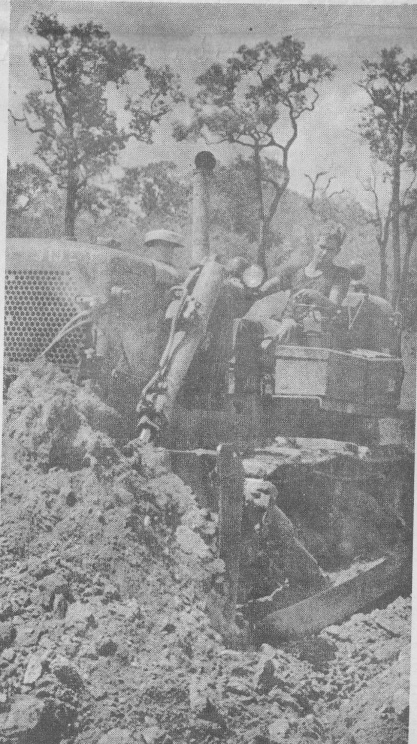
Specialist 4 William Aaron pushes up the berm of Fire Support Base Wilma.
